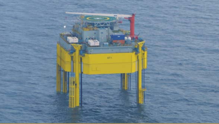
Transformer station built by ALSTOM is set up 22m above water
